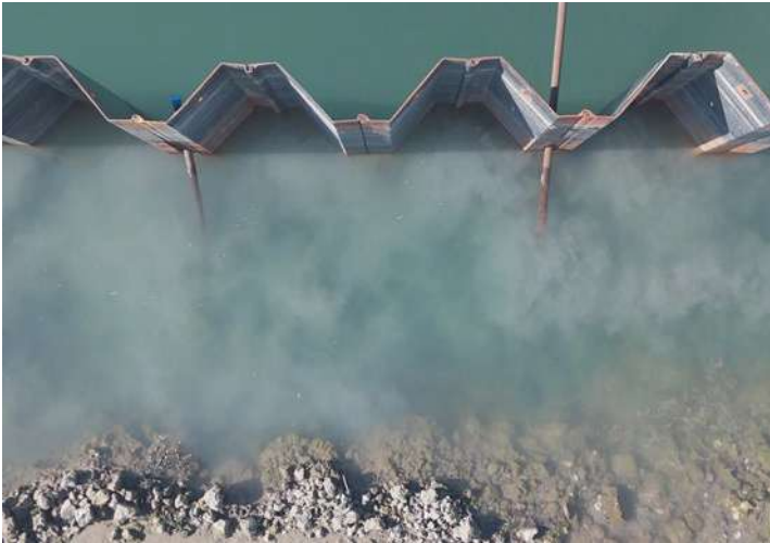
Carbon-storing port infrastructure (Paebbl)
