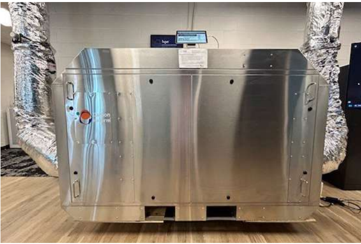
HVAC-connected Carbon Capsule (Carbon Reform)
